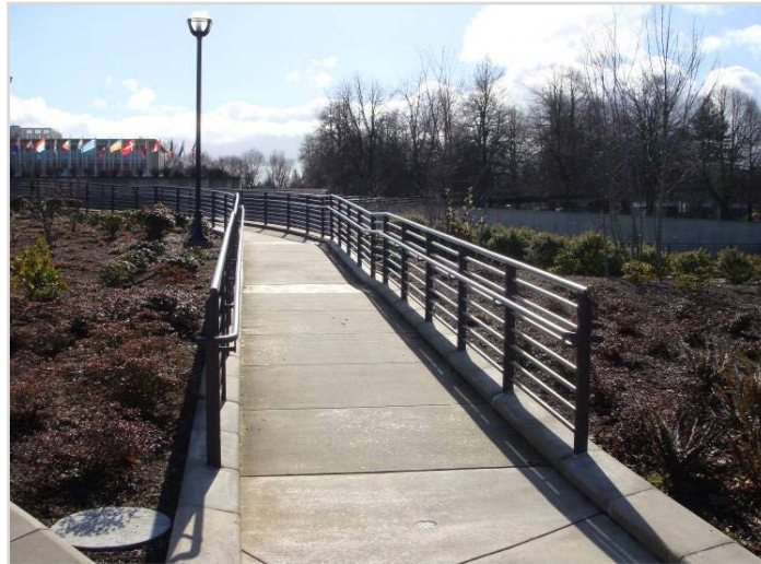
Access Ramp With Accessible Handrails Exhibit 1510-30
