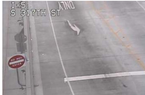
Do Not Enter sign located on the left side at the top of each off-ramp.
