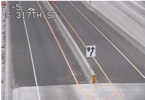
Keep Right sign located at the top of the median barrier separating on- and off-ramps.
