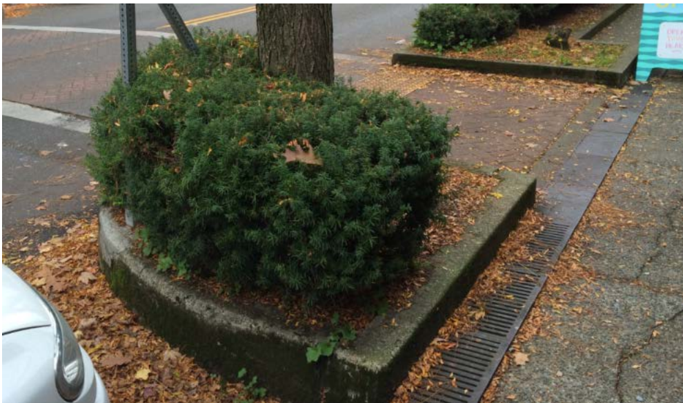
Downtown City of Olympia 5th Avenue Curb Retrofit. Note that retrofits like this must comply with 1510.07(1)(c) , see Chapter 1510 .
