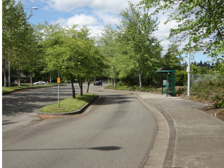
Bus Pullout with Longitudinal Island
