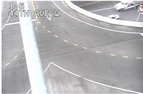
Guide striping provided for left-hand turns.
