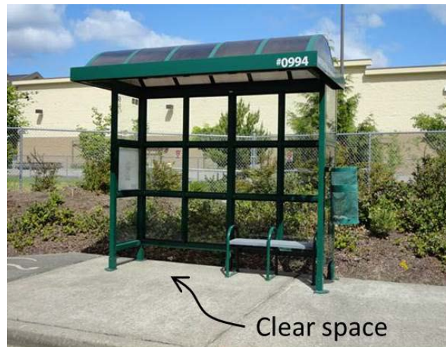
Passenger shelter showing clear space
