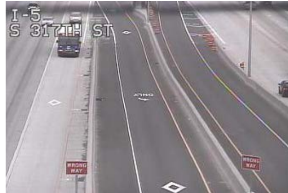
Diamonds and Turn Only pavement markings on off-ramps.
