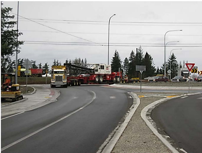
Roundabout showing colored truck apron at central island and at buffer area between travel lanes and sidewalk
