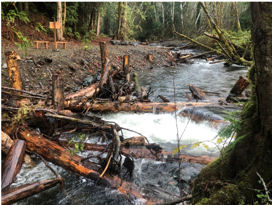
Figure 10-4 Example of Small-Channel Complex Log Grade Control
