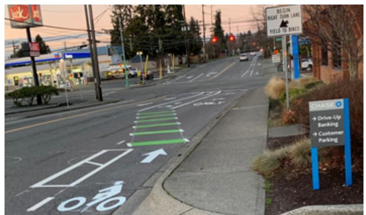
City of Tacoma's Trail to Transit Connector uses new pavement striping to connect bike lanes on S. Mildred Street.
