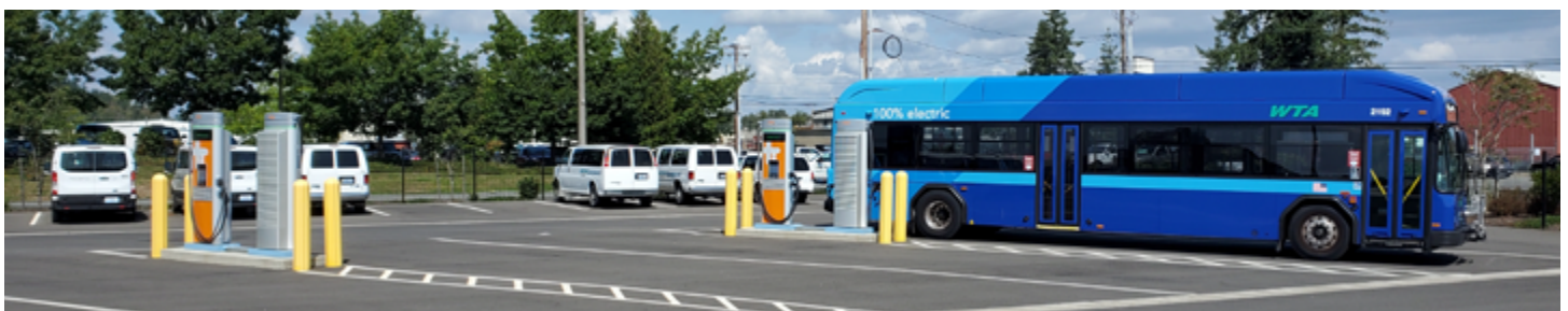
Whatcom Transit Authority worked with Puget Sound Energy on the design of a new bus yard that includes electric bus charging stations.
