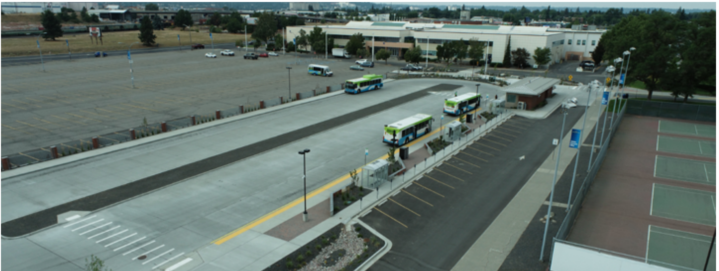
Spokane Transit's relocated and expanded Spokane Community College Transit Center provides enhanced customer amenities and improved rider safety.
