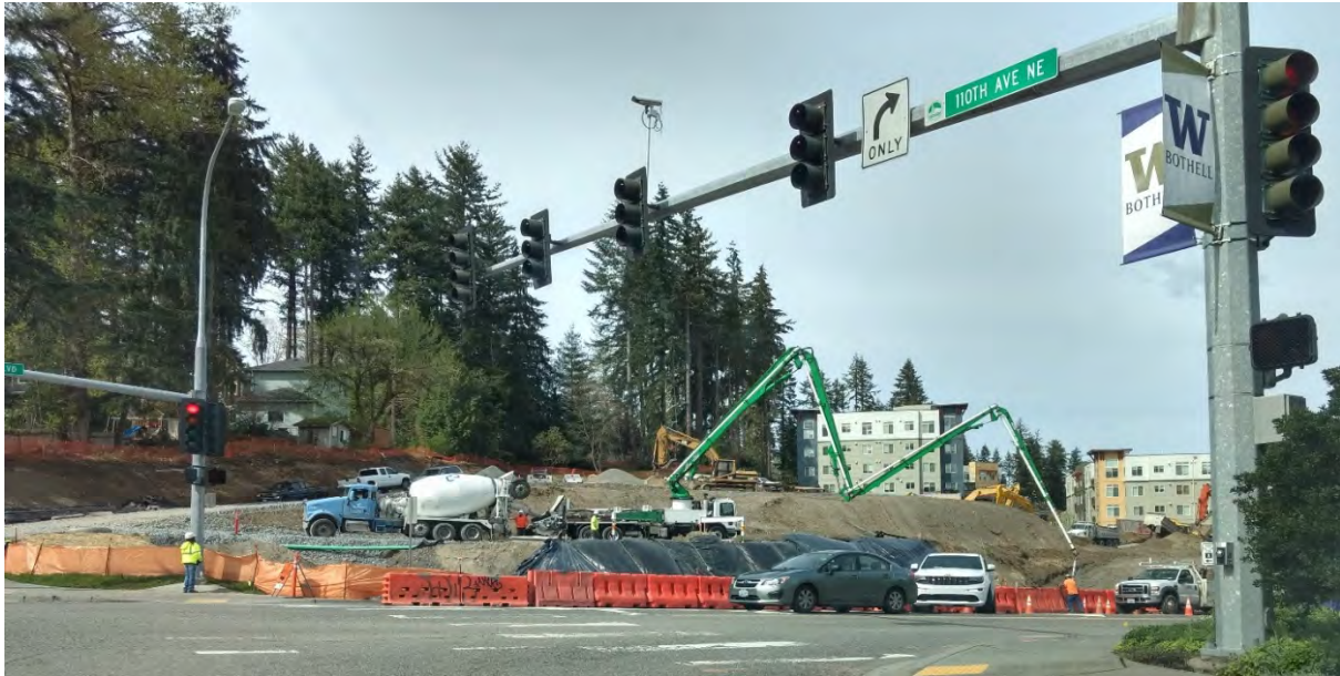
Photograph 7 – View of new construction of Beardslee South Townhouses, looking north.
