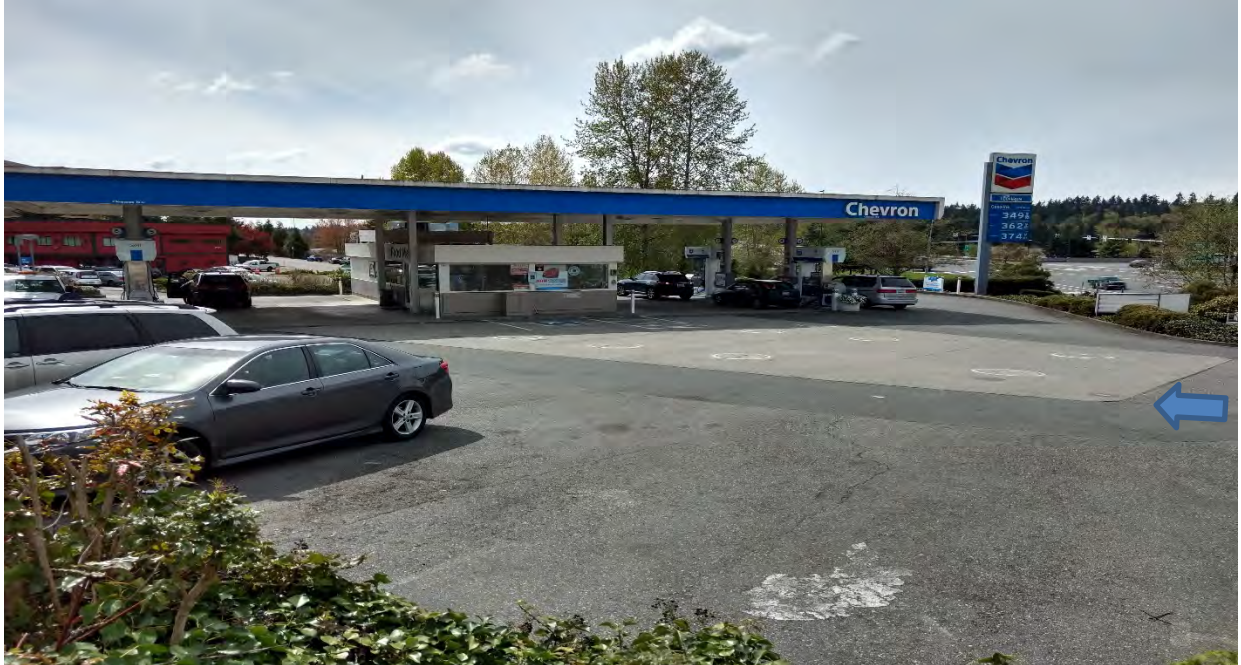
Photograph 1 – View of Chevron 93299 cleanup site at 15900 116th Avenue NE, Bothell, looking west. Note monitoring well monument.
