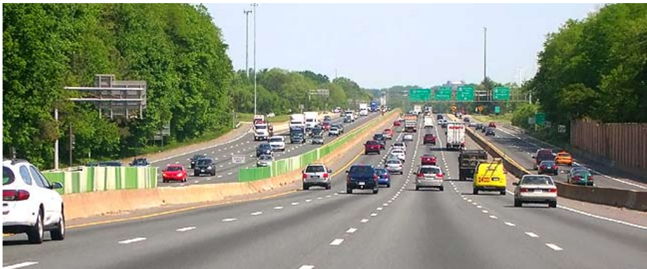
I-495 Capital Beltway in Virginia.
