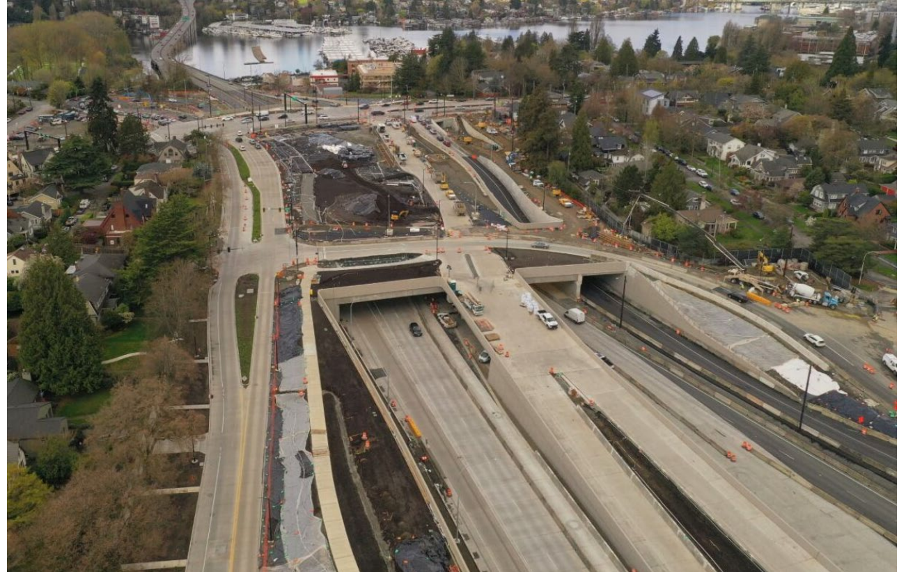
HOV direct access ramps (March 26)
