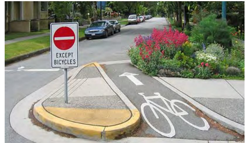
Bicycle connection through a channelization island with a do not enter except bicycles sign.
