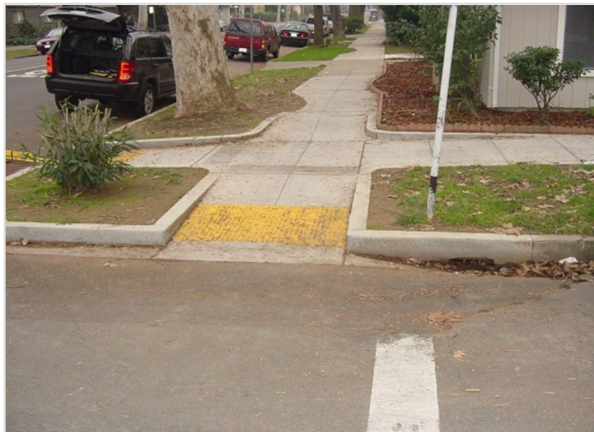
Combination Curb Ramps Exhibit 1510-13
