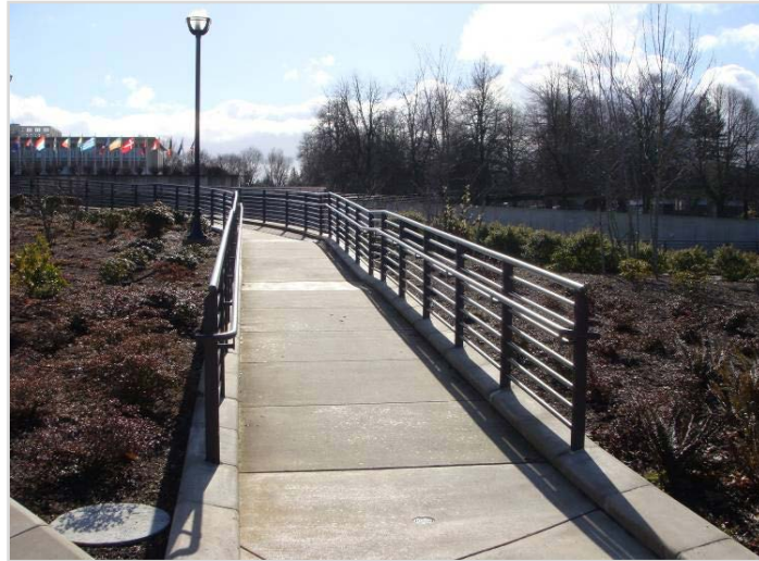
Access Ramp With Accessible Handrails Exhibit 1510-30
