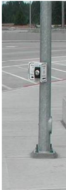
Typical Pedestrian Pushbutton Exhibit 1510-23
