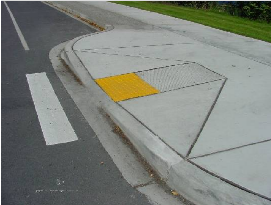
Perpendicular Curb Ramp Exhibit 1510-9
