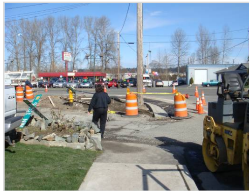
Does not meet ADA requirements
