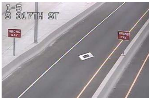
Wrong Way signs (30° rotation at potential wrong-way entrance point).
