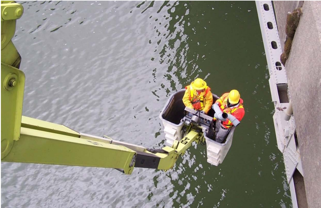
Cleaning bridge drains requires special equipment and traffic control
