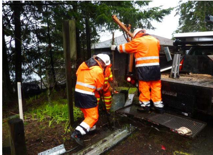
Replacing a guardrail is not a simple activity
