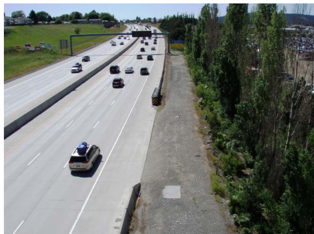
Ideal utility vault and Variable Message Sign access
