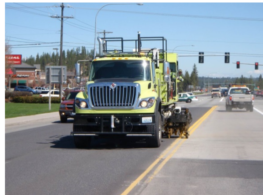
Striping crew restriping after patching pavement
