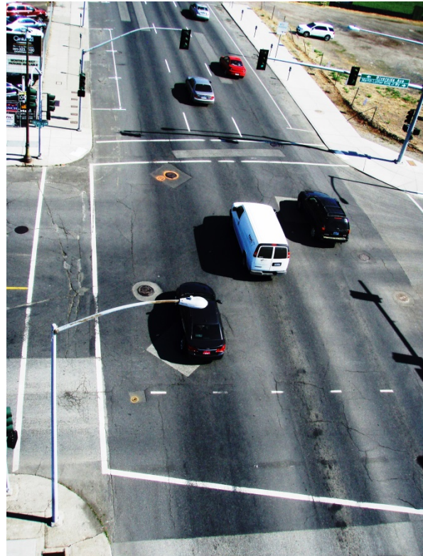
Poor utility vault access
