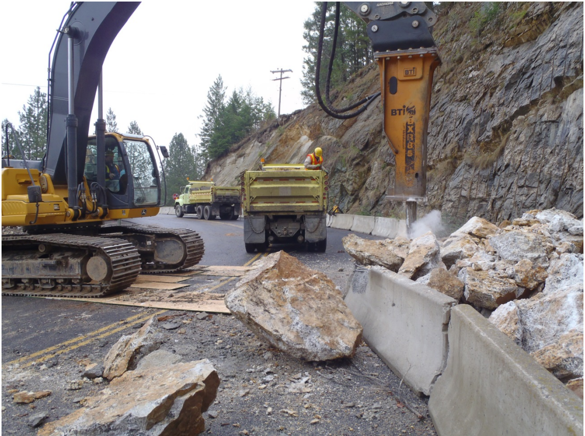
Maintenance clearing highway from rockfall overburdening catchment area
