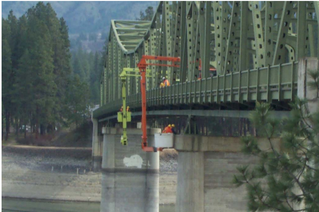
Figure 1 Typical multi-crew UBIT inspection
