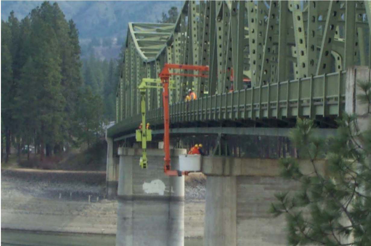
Figure 1 Typical multi-crew UBIT inspection
