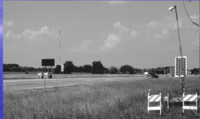
Illinois DOT I-55 Bridge Construction Real Time Work Zone Traffic control system
