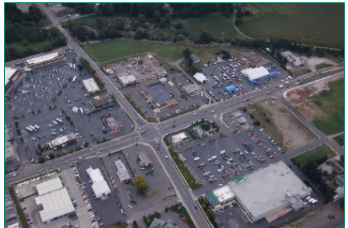
SR 539 at Kok Road where segment narrows to two lanes.
