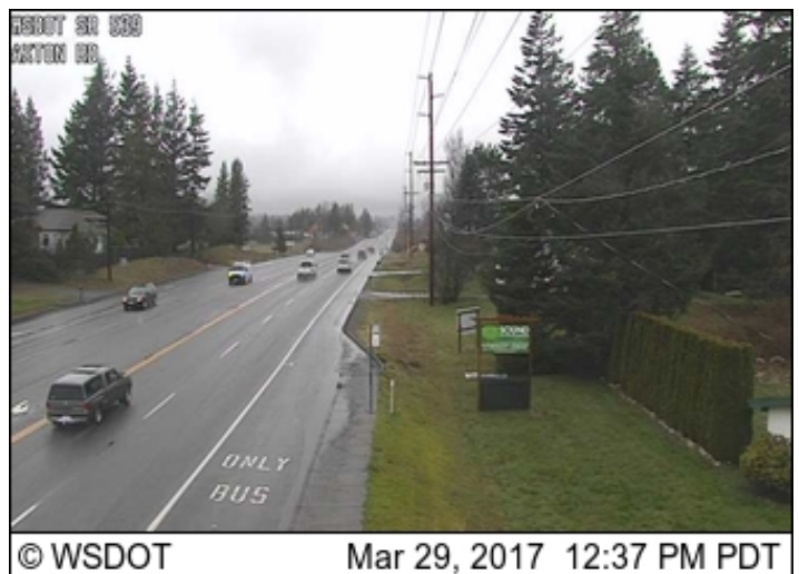
A transit stop on SR 539 with a bus pullout.
