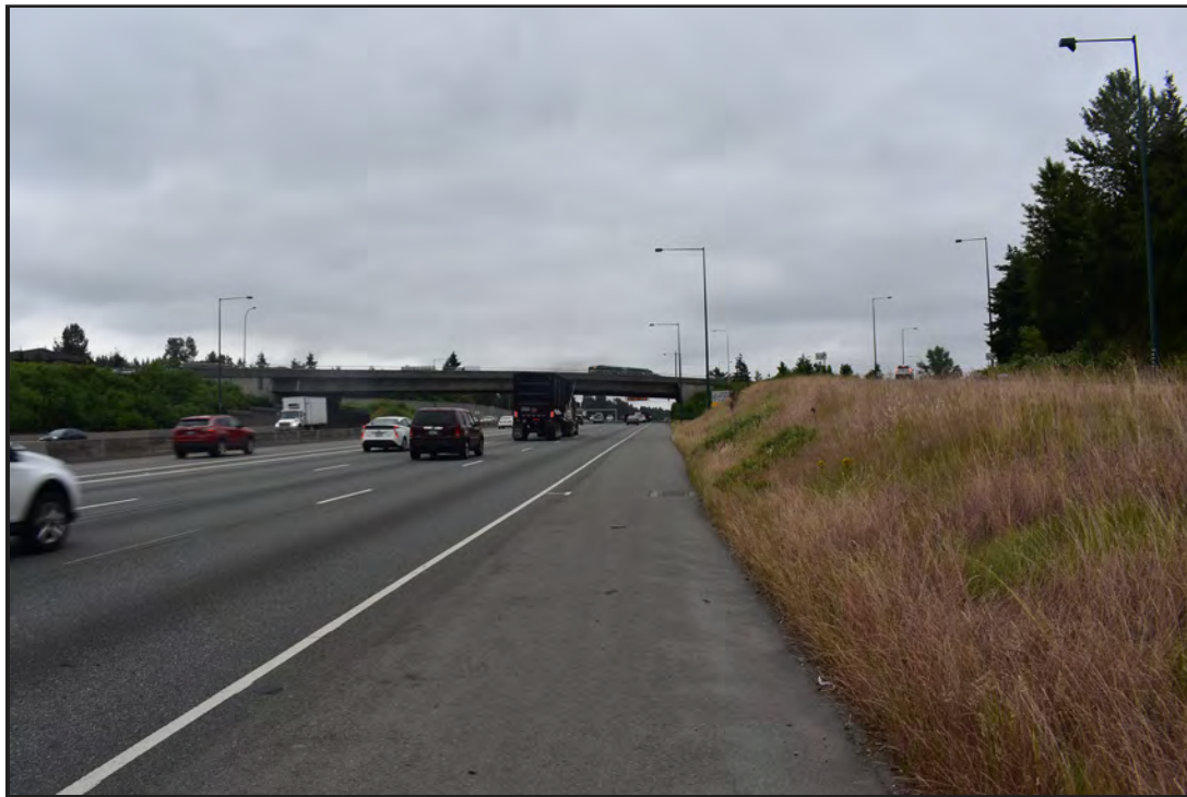
Exhibit 6-8. Overview of Zone 17 in the southern project study area, view is to the north.
