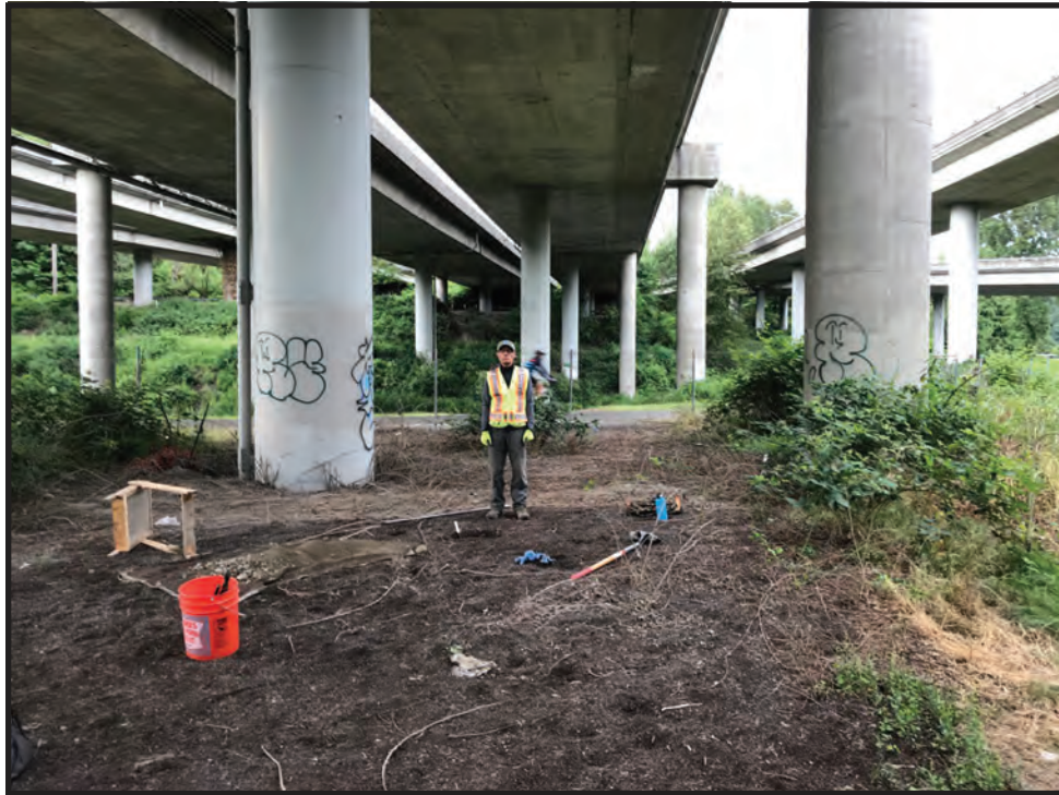
Exhibit 6-19. Overview of the I-405/SR-522 interchange area near the southern boundary of Zone 19, view is to the south. This modified landscape contains numerous overpass supports and significant sediment disturbances. Crewmember is standing at ST 27 with the Sammamish River and bike trail in the background.
