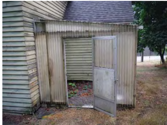
Shed addition, facing west
