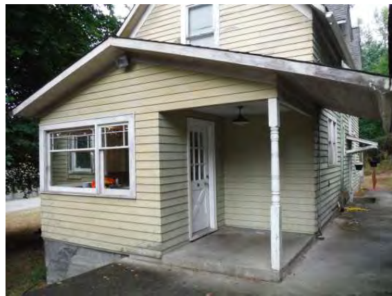
Stoop detail facing southwest
