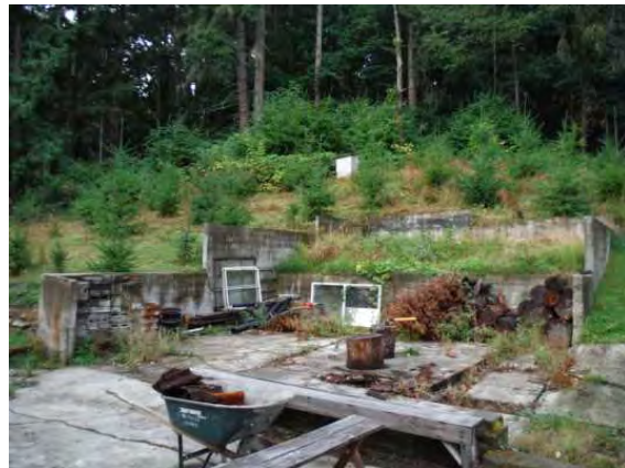
Demolished garage, facing southwest
