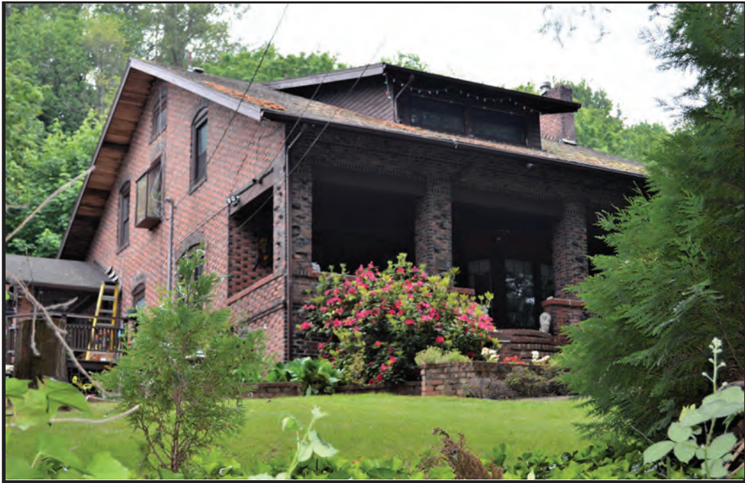
Exhibit 6-17. Constructed in 1906, property 40731 is an excellent local example of Craftsman/Bungalow style architecture, view is to the south. The brick dwelling maintains good integrity, and was determined eligible by DAHP for listing in the NRHP in 2005. The project will not impact the historic property.
