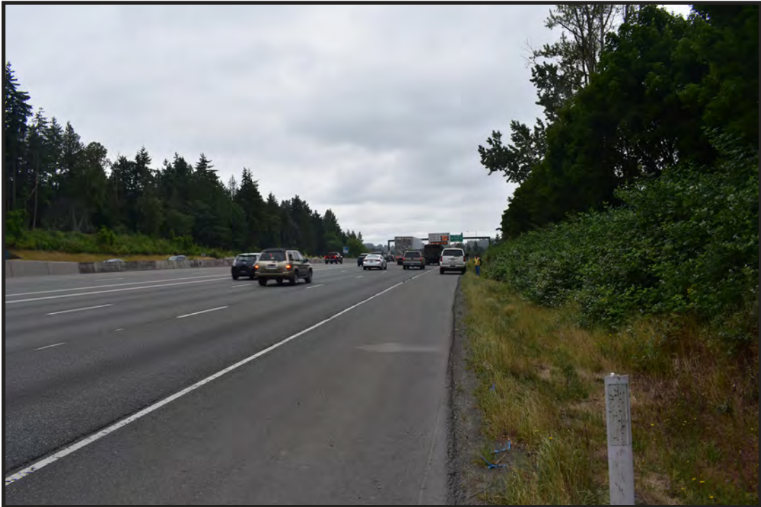
Exhibit 6-4. Overview of Zone 15 in the southern project study area, view is to the south.
