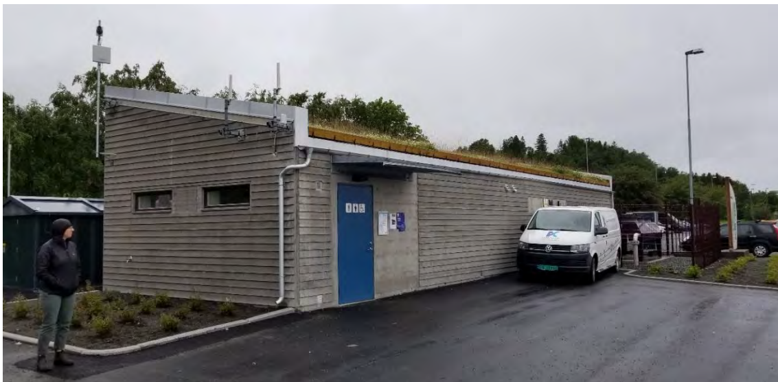
Figure 6: Shoreside Battery Bank in Flakk, Norway
