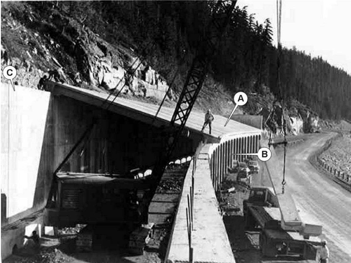
Exhibit 5-4 Lake Keechelus Snowshed Bridge Construction in 1951
