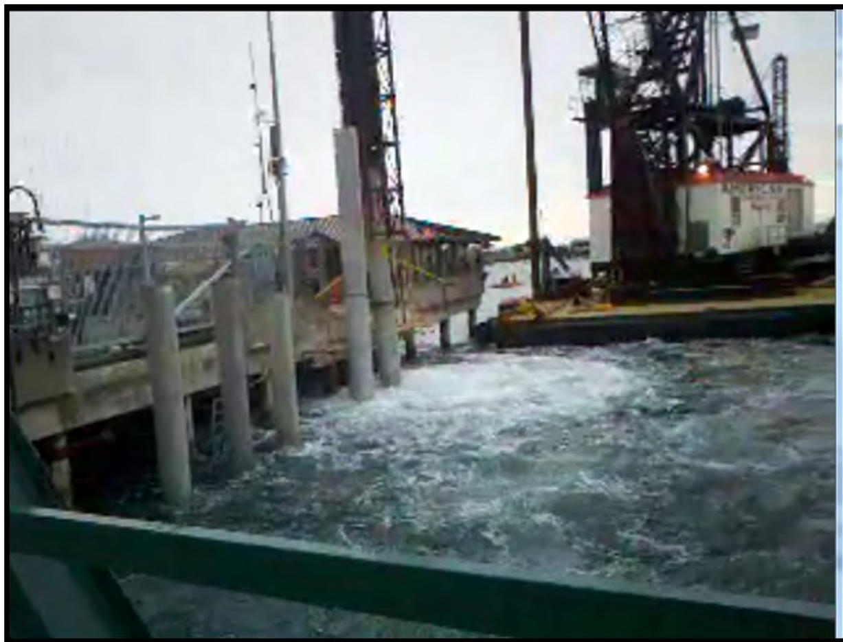
Figure 6: Impact Pile Drive with Bubble Curtain.
