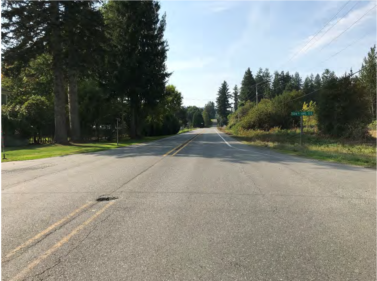
Figure 4.2.4 – SR 202 Intersection with 324th Avenue Southeast
