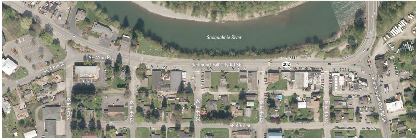
Figure 4.2.1 – Overview of SR 202 in Fall City
