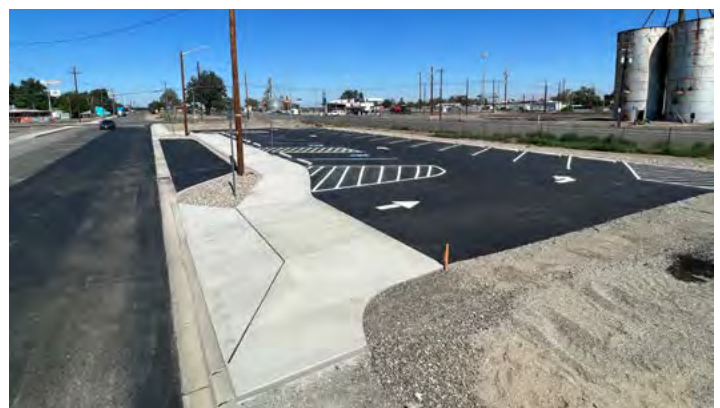
Modernization underway at Mabton’s park and ride.
