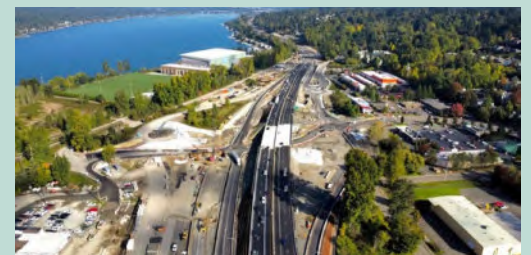
Aerial view of Renton to Bellevue Project work during summer 2023.
