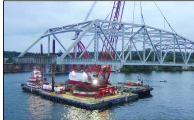
A derrick barge removes a metal truss from the old SR 520 floating bridge.
