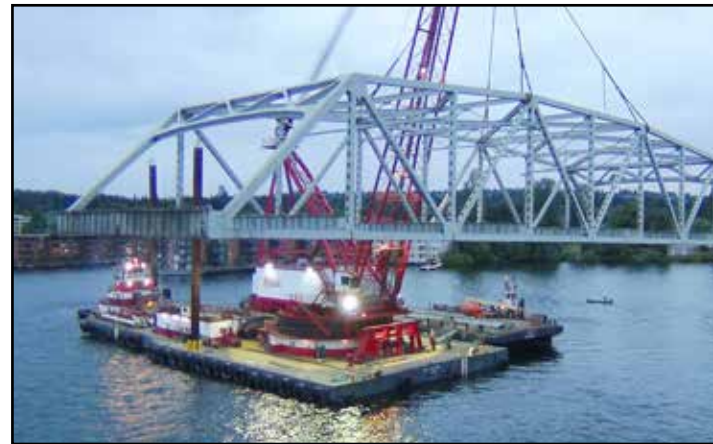
A derrick barge removes a metal truss from the old SR 520 floating bridge.
