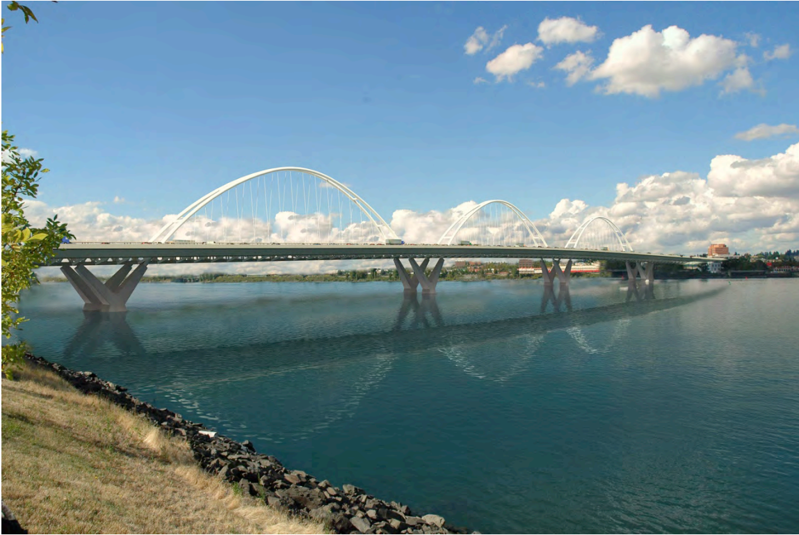
Figure 18 – Riverbank View of Tied Arch Bridge
