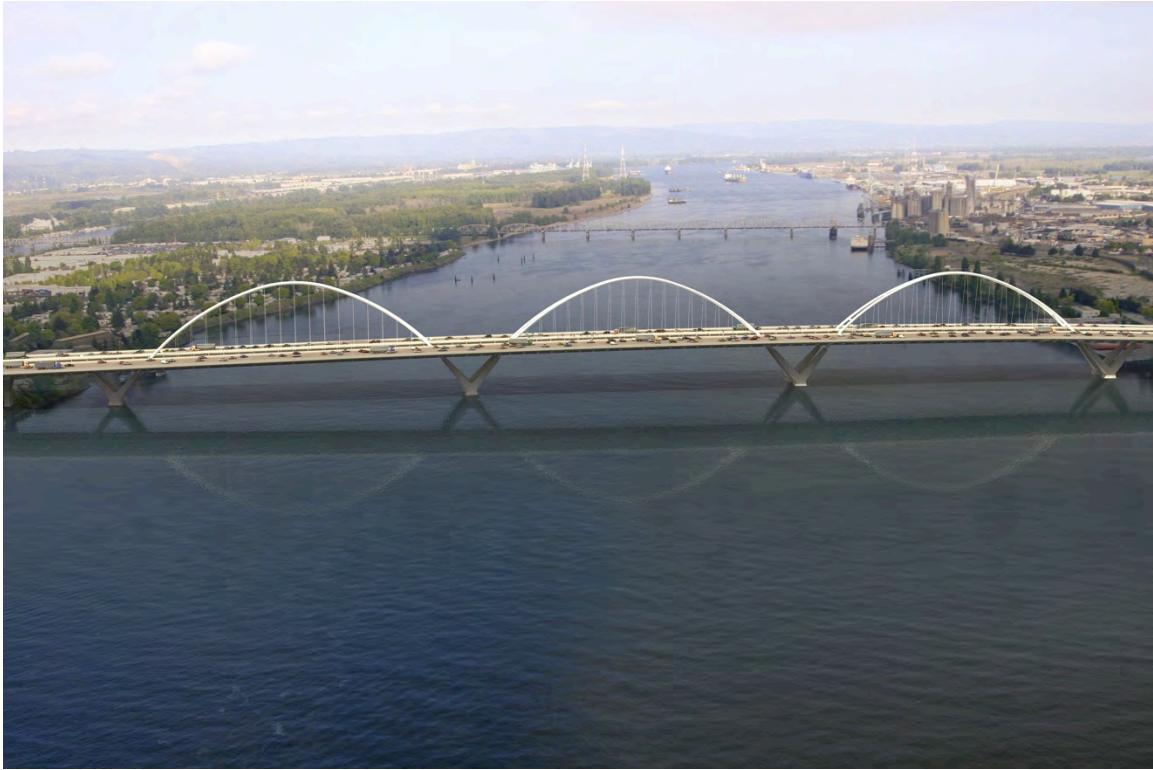
Figure 13 – Aerial View of Tied Arch Bridge
