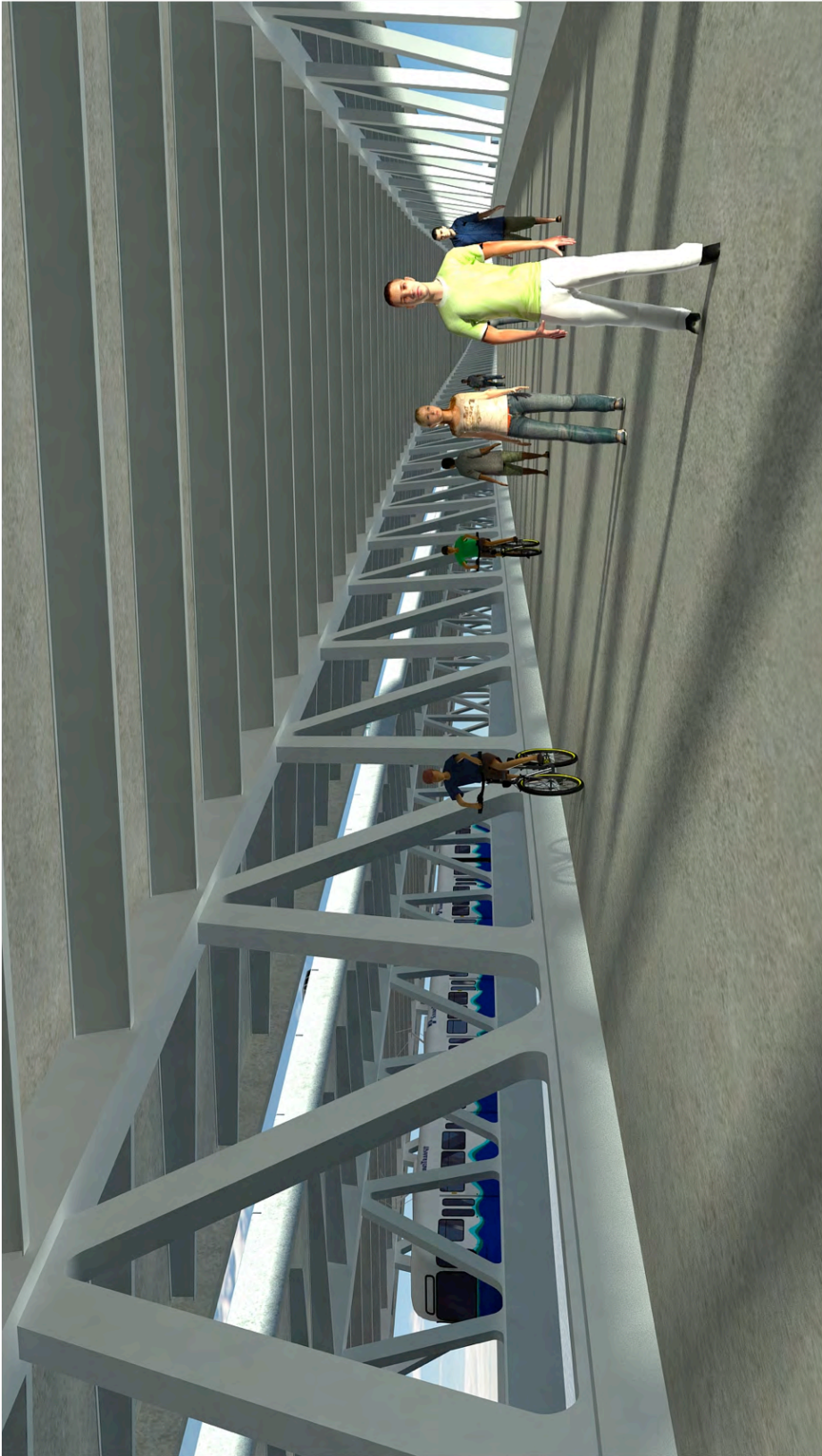
Figure 35 – Multi-Use Path View of Composite Deck Truss Bridge
