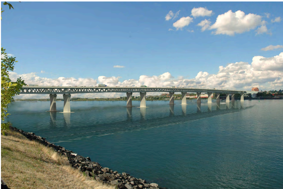
Figure 30 – Riverbank View of Composite Deck Truss
