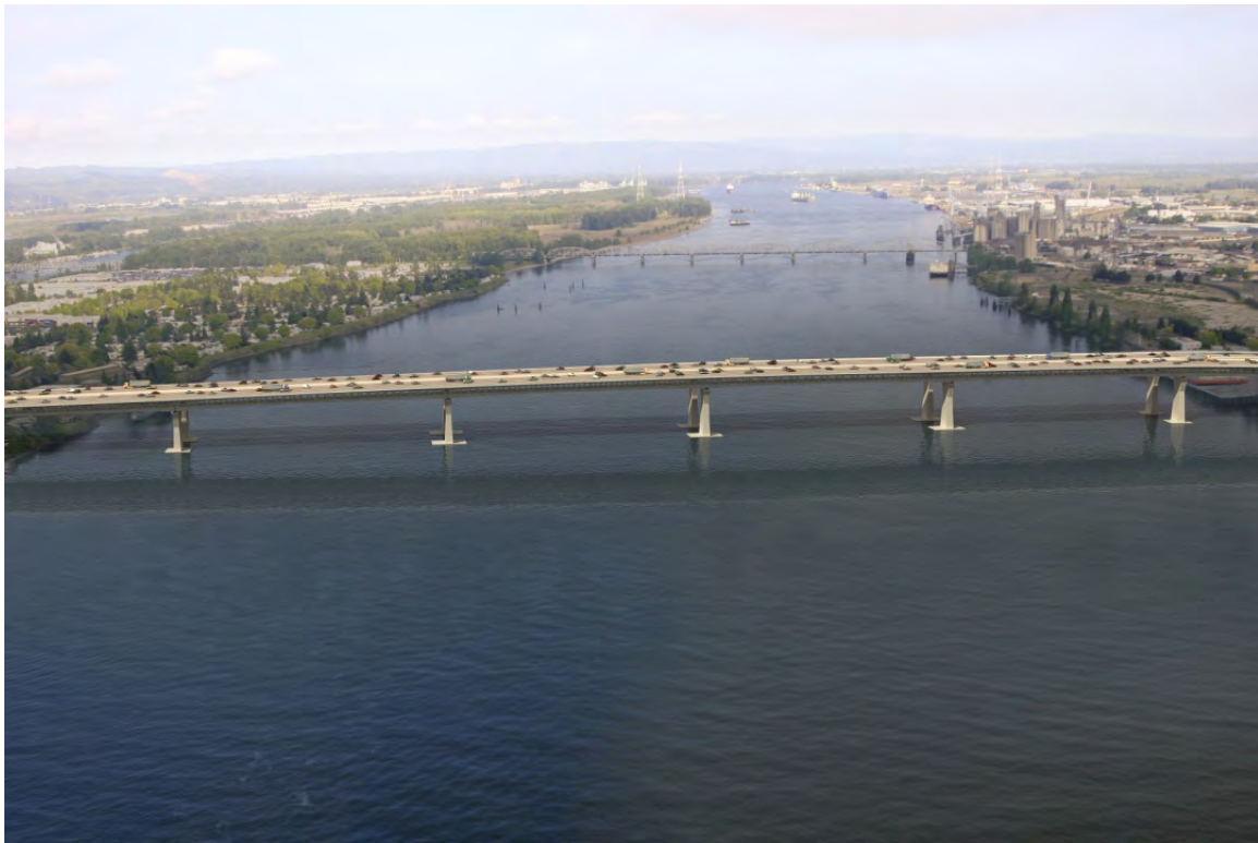
Figure 23 – Aerial View of Composite Deck Truss Bridge
