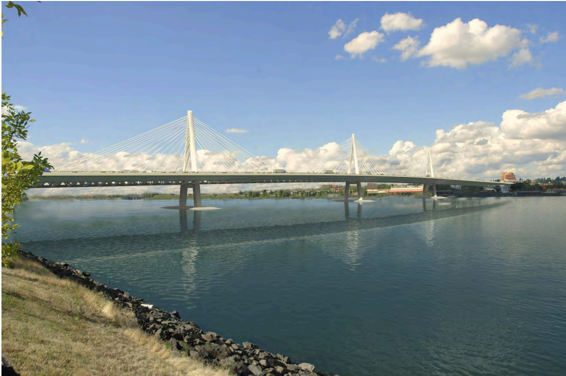
Figure 7 – Riverbank View of Cable-Stayed Bridge
