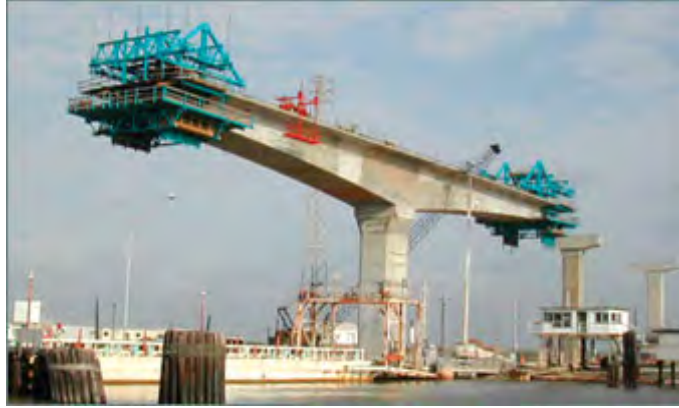
Figure 45 – Cantilever Construction, Cast-in-Place with Form Travelers
