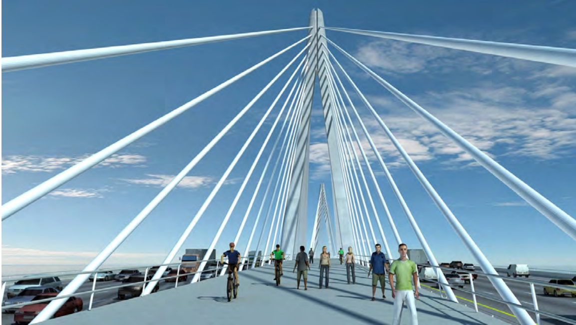
Figure 9 – Multi-Use Path View of Cable Stayed Bridge
