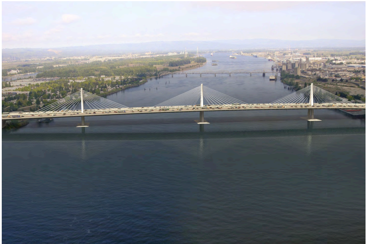
Figure 2 – Aerial View of Cable-Stayed Bridge
