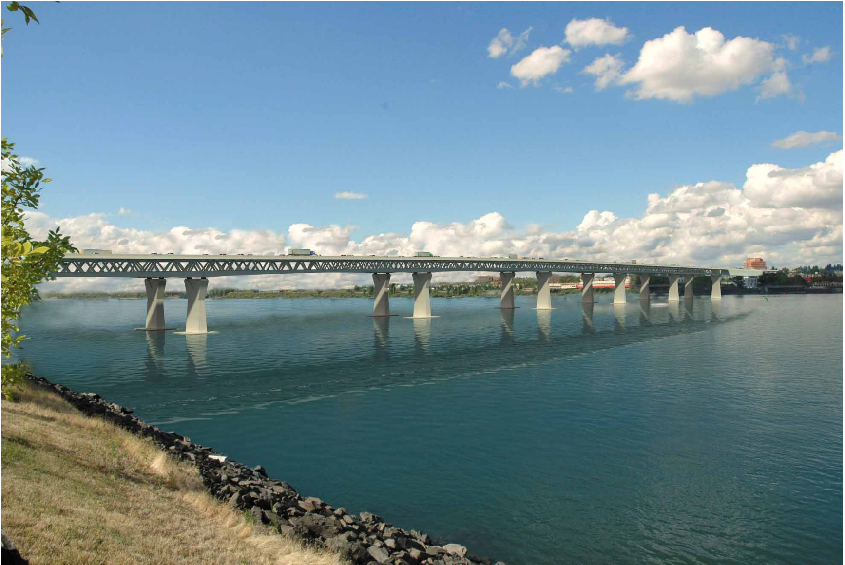
Deck Truss Bridge Type | Looking north to Vancouver
