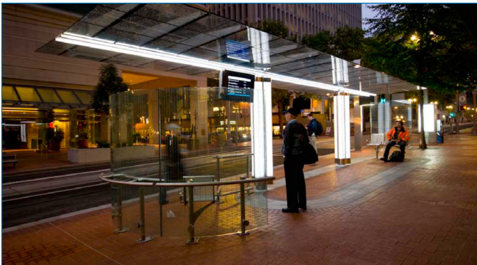
Station lighting increases visibility for those on or approaching platforms.
