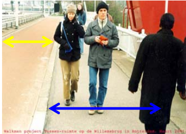
Willemsbrug Rotterdam, Netherlands 6' sidewalks (2) 6' bike lanes (2) Total: 24'
