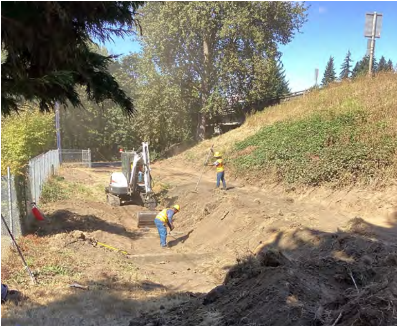
Figure 4. Southwest Region Area 1 crew reconstruct a bioswale in need of maintenance.
