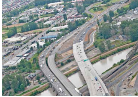
The new northbound I-5 bridge over the Puyallup River is finished and open to all traffic.
