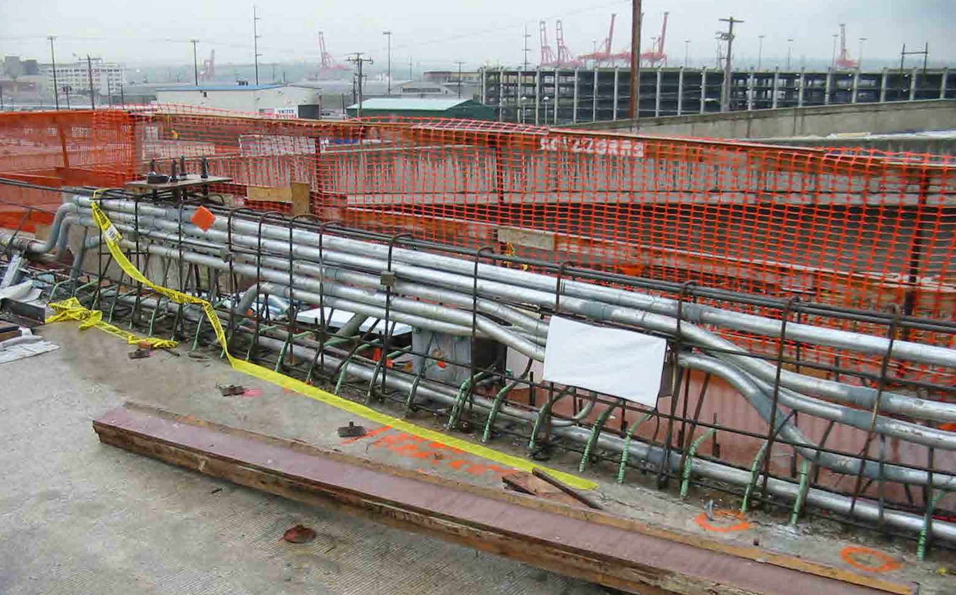
Conduit in Bridge Rail
