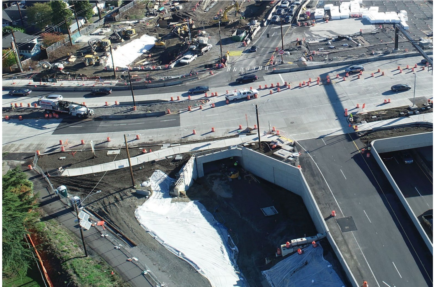
West entrance to the tunnel under Montlake Boulevard (Oct. 18)
